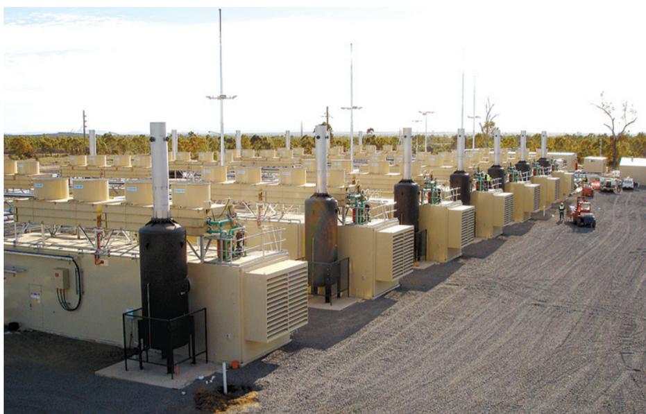
Above: Jenbacher engines located on the 15 x 64m<sup>2</sup> engine bases
