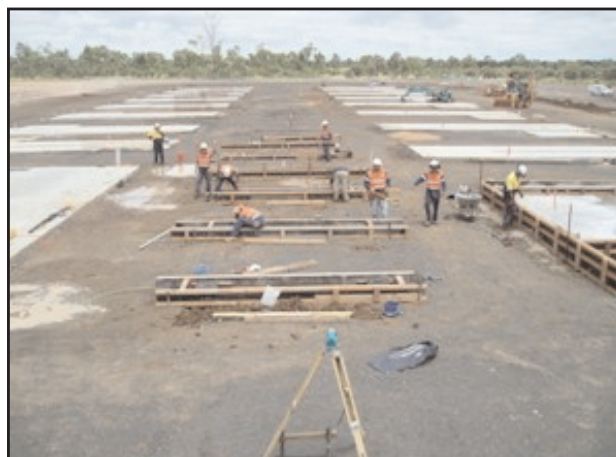
CONCRETE SLABS FOR POWER STATION — MORANBAH NORTH
