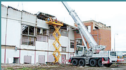
BUSBY DEMOLITION Ray Busby - Ph: 0408 883 654
