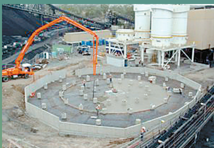
BUSBY CONTRACTORS Patrick Busby - Managing Director, Project Manager, Civil Engineer Ph: 0418 727 495
